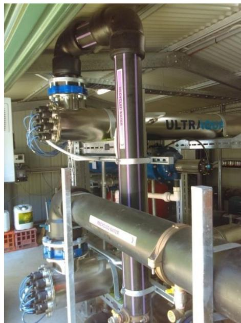
Figure 4 Two new UV Disinfection Units Installed in Cammeray Treatment Shed
