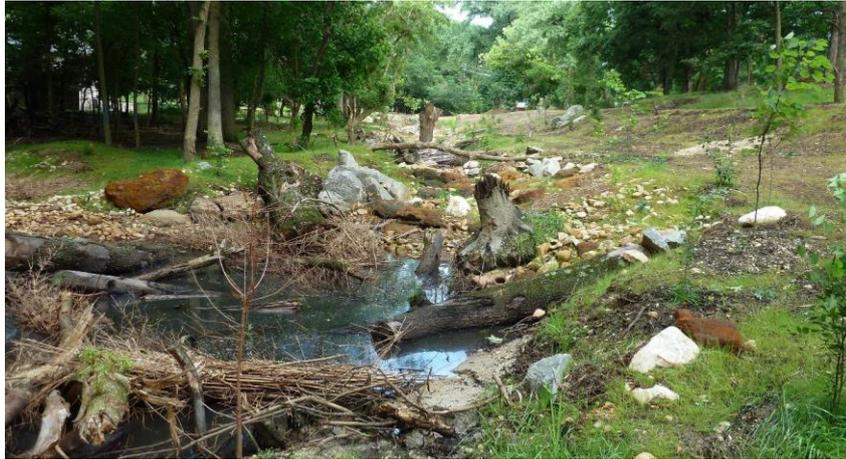
**Figure 8: Example of large woody debris integrated into an urban stream restoration project.**
