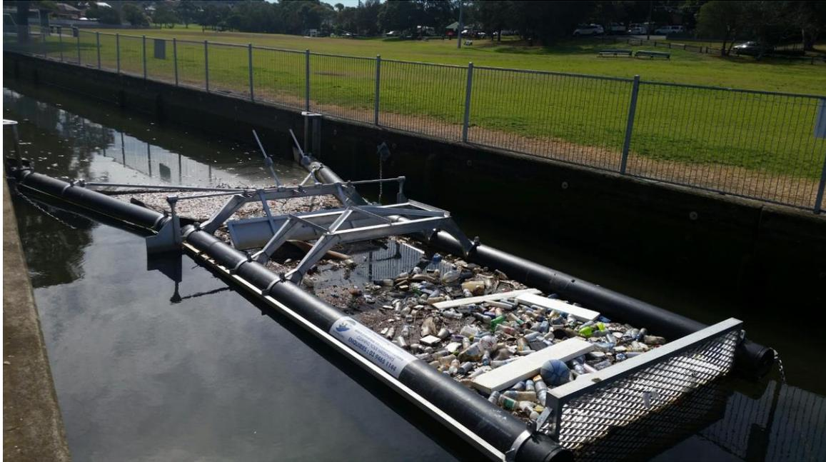
Figure 2. Kogarah Bay Creek litter boom. One of six booms installed as early parts of the program
